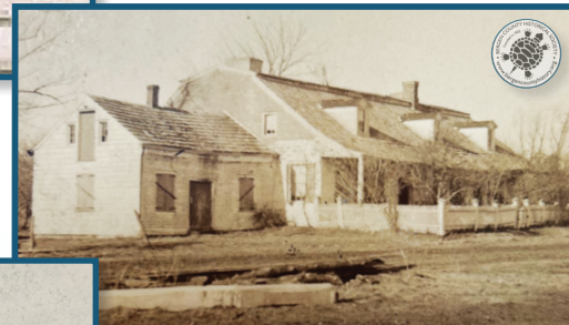
PIC 3 DAVID ANDERSON ZABRISKIE IS PICTURED IN A 1908 PHOTOGRAPH OF THE ZABRISKIE-STEUBEN HOUSE WITH A WRAP-AROUND PORCH, AN ATTACHED KITCHEN, AND FOUR DORMERS. NOTE THE DATE STONE.
